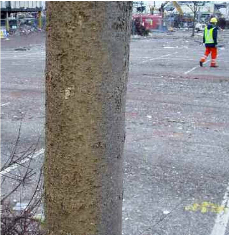
Figure 17 Abrasions to the base of a tree in the Northgate building west car park, viewed from the south
