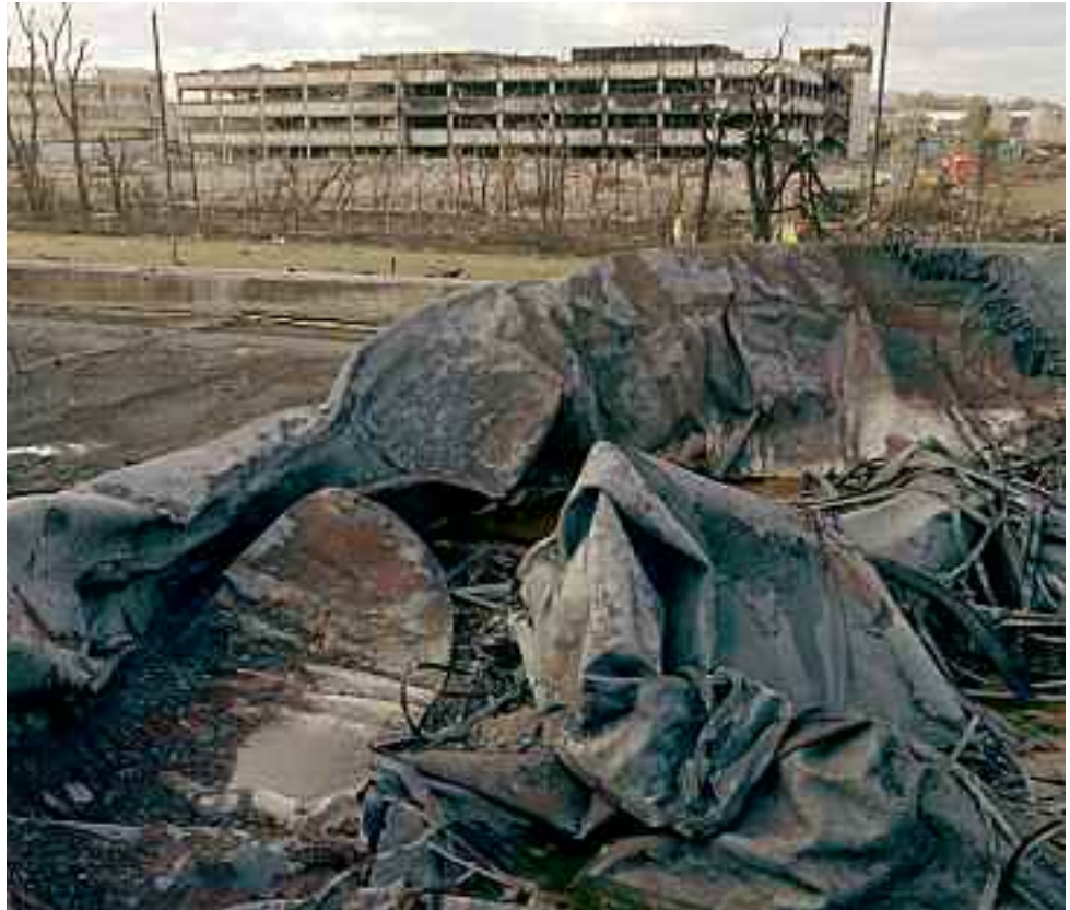
Figure 10 Looking south-west towards the Northgate building from Tank 915 (HOSL West)
