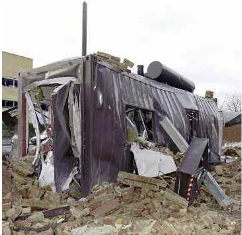
Figure 21 Emergency generator cabin, close to the south-east corner of the Northgate building, viewed from the north east. The north-east segment of the damaged 3-Com building is shown to the left of the picture
