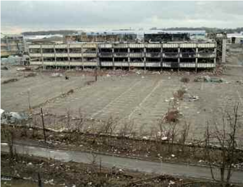
Figure 8 Looking west into Northgate building car park, from the position of Tank 912 (HOSL West)
