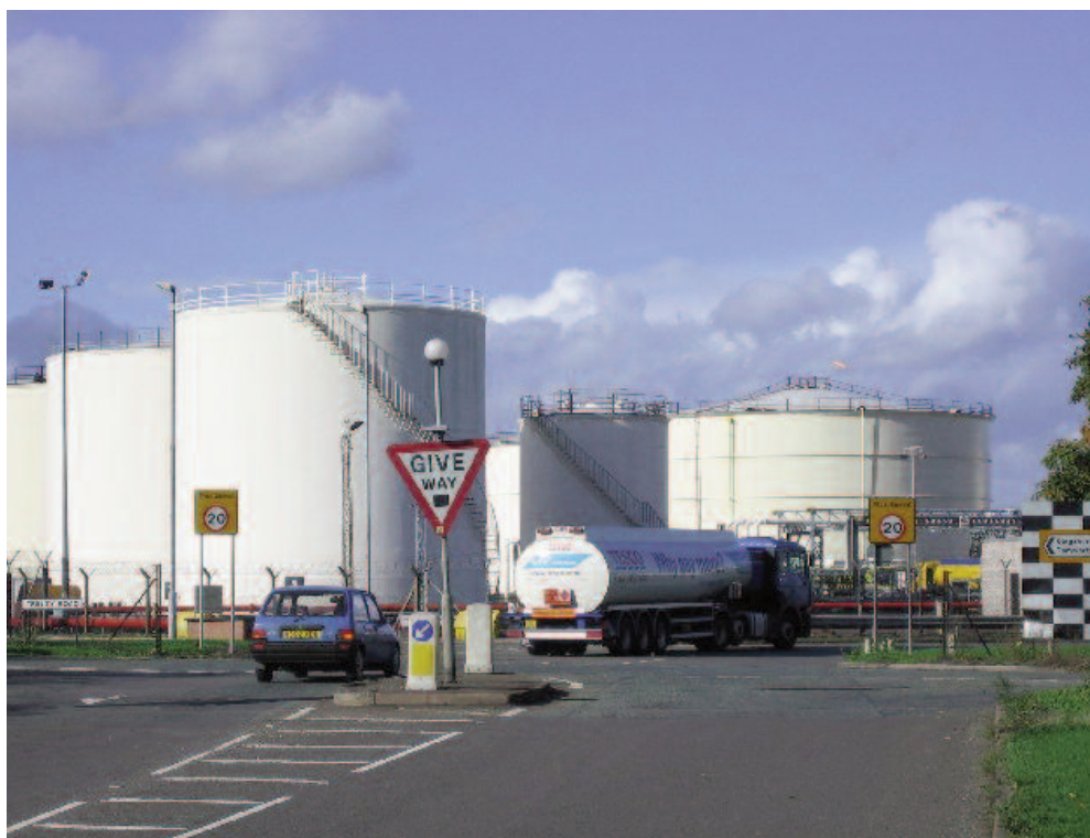
Figure 15 A view of the Kingsbury fuel storage depot in Warwickshire. Kingsbury is a facility of a similar size and function to Buncefield
