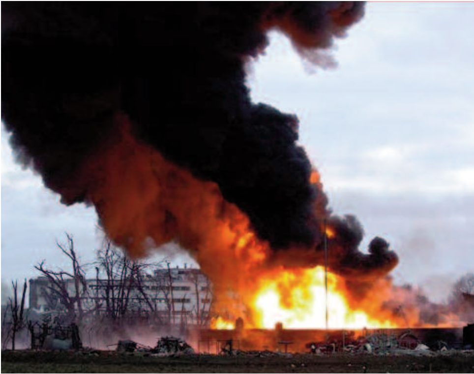
Figure 19 The remains of the fire in Tank 12 at Buncefield, on the BPA depot. This was the largest tank on the Buncefield site and could store 19 million litres of aviation fuel
