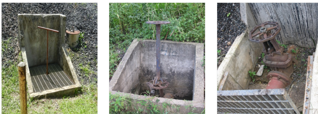
Figure 15: Various dike drain valves at CAPECO. Tank 409 fixed stem dike drain valve (left): position of the valve is undeterminable without physically turning the valve. Rising stem valves (center, right). In some cases, the valve position is hidden in the sump (center).
