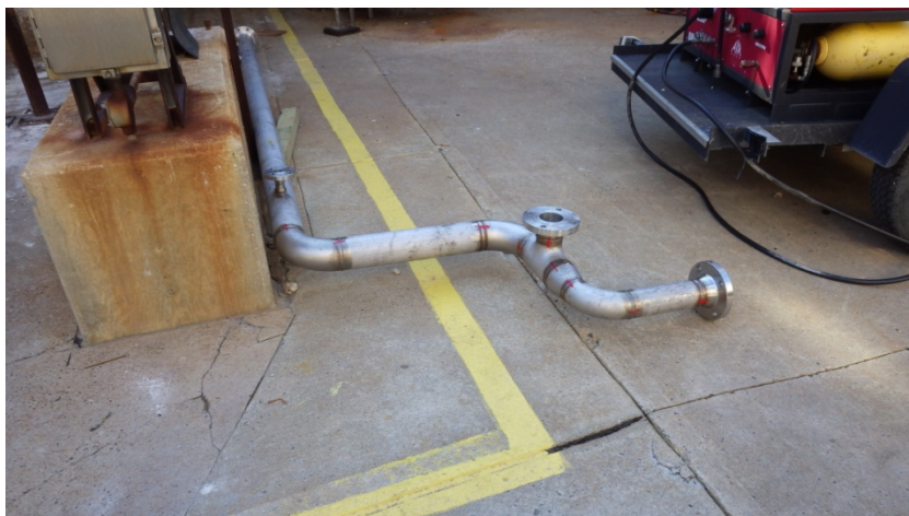
FIGURE 2. 20-foot replacement piping (Source: CSB).
